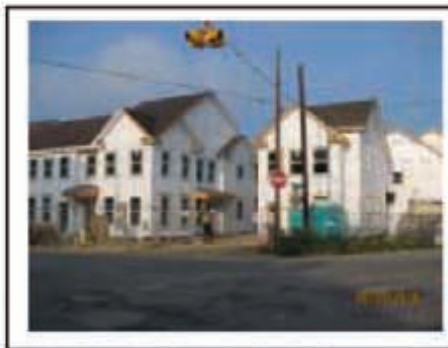
35th & Jacobin Street (Under Construction)
