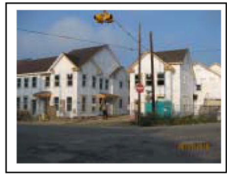
35th & Jacobin Street (Under Construction)
